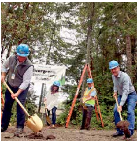
PSD gets to work on the first new elementary school on the Key Peninsula in a generation.
